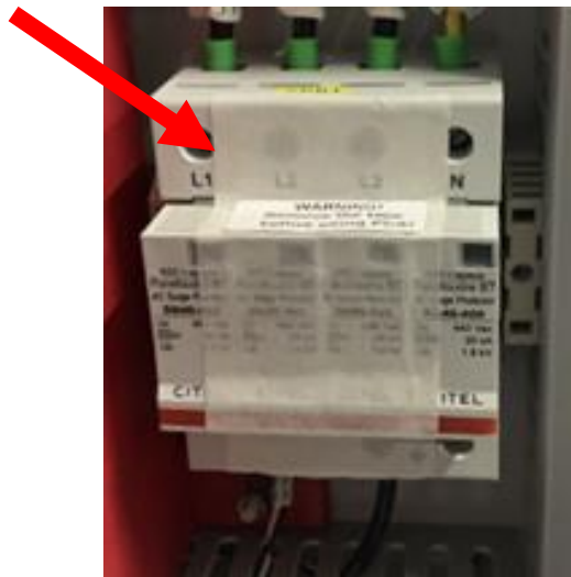
Figure 41. Remove the adhesive tape on AC SPD
