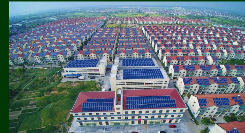
Project "Million Rooftops for Zhixi" 4MW | Quzhou, Zhejiang Province, China
