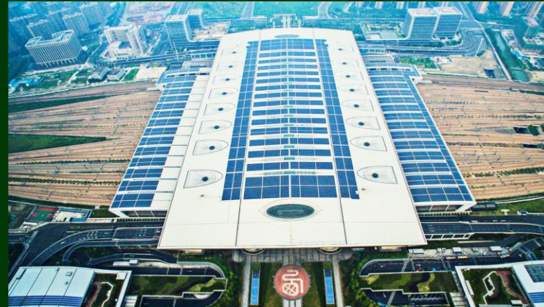
Roof Photovoltaic Power Station of Hangzhou East Railway Station 10MW | Hangzhou, Zhejiang Province, China
