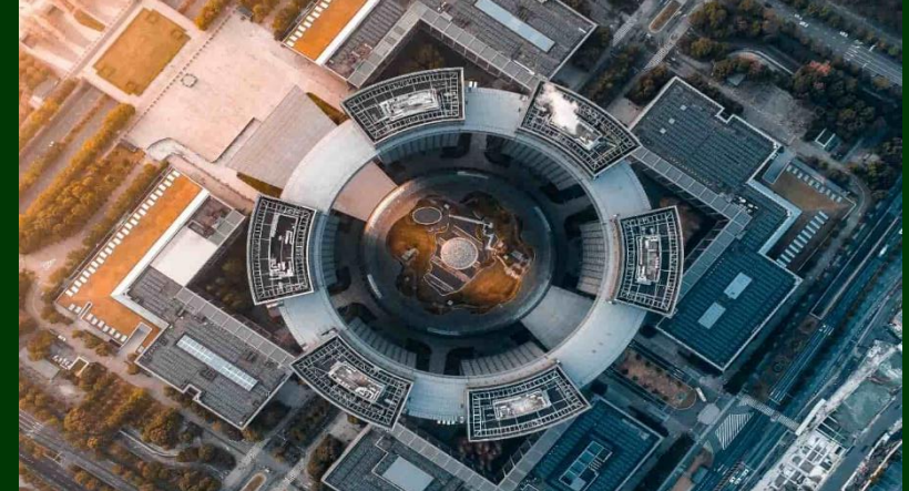
Hangzhou Civic Center Podium Roof Photovoltaic Power Station 1.2MW | Hangzhou, Zhejiang Province, China
