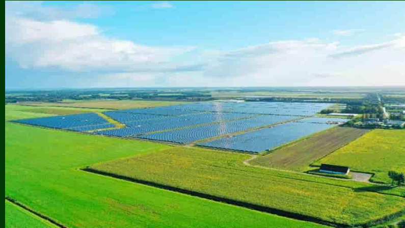
Midden-Groningen Solar Park, one of the Largest Power Stations in the Netherlands 103MW | The Netherlands
