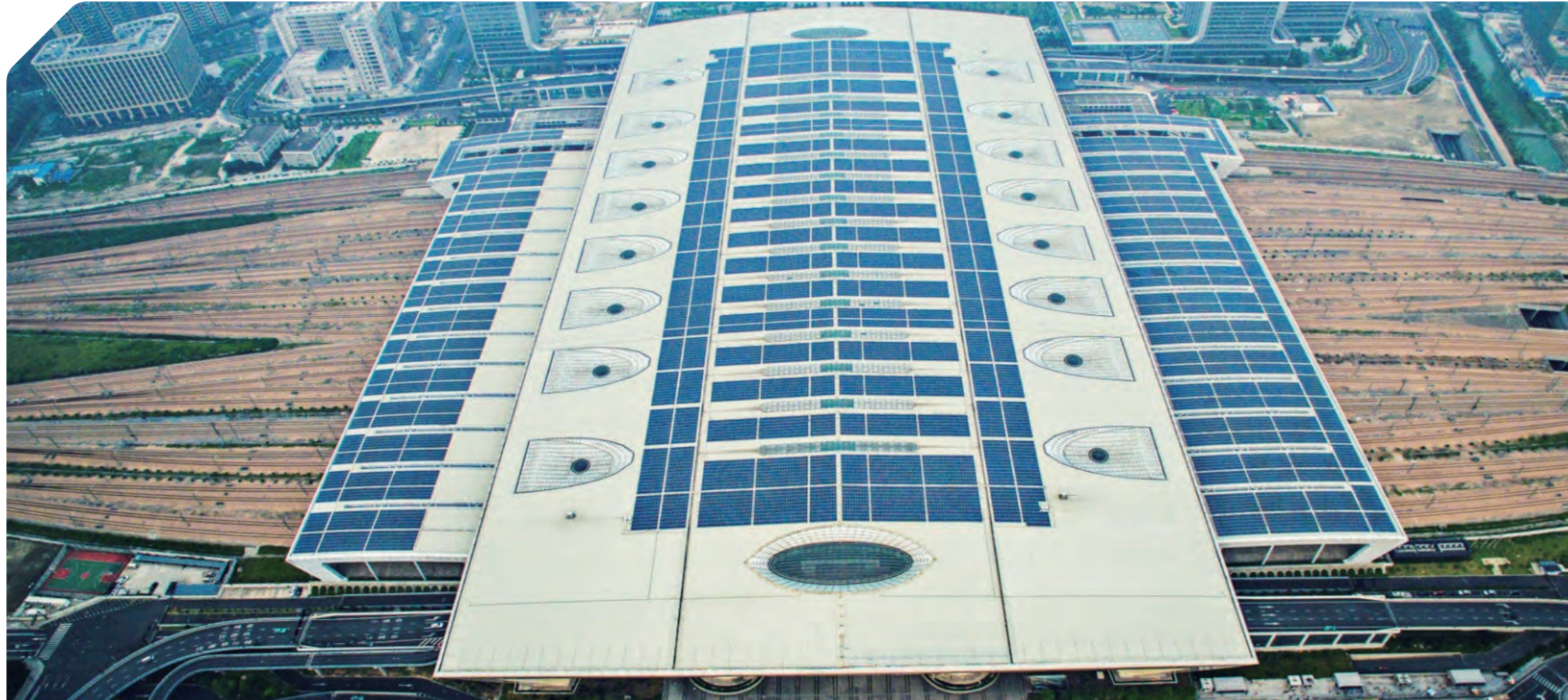
10MW Roof Photovoltaic Power Station of Hangzhou East Railway Station Hangzhou, Zhejiang Province, China
