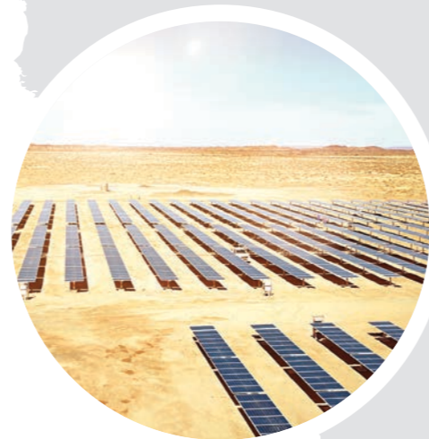
KEETMANSHOOP, NAMIBIA Power generation: 6 MW
