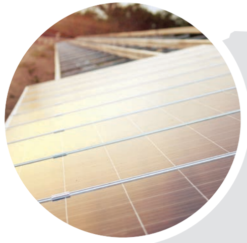
1. NORMANTON SOLAR FARM, QLD Module: CS6X-P Power generation: 5 MW
