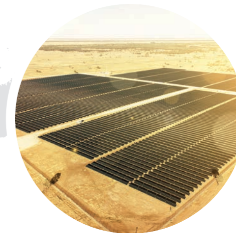
LONGREACH, AUSTRALIA Power generation: 17.4 MW
