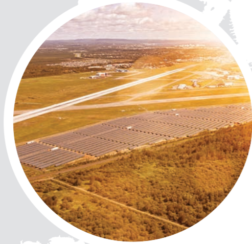
THUNDERBAY AIRPORT, CANADA Power generation: 8.5 MW
